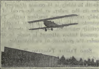
Taking unnecessary chances. Gliding over buildings for landing with insufficient clearance.
